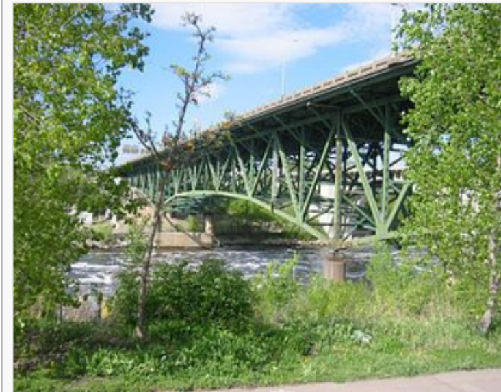
Bridge 9340 in May 2006
