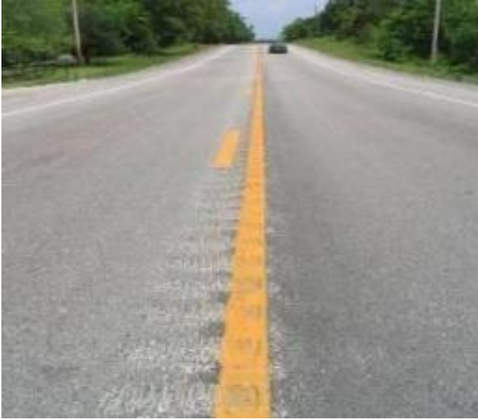
Centerline Rumble Strip
